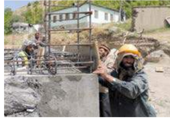
Local masons were taught to build earthquake resistant houses.
