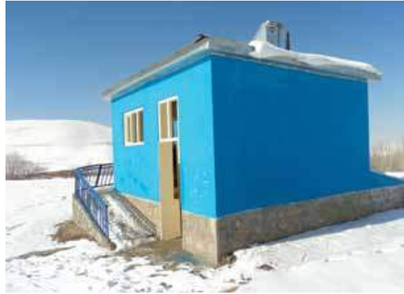
Latrine constructed by NAC in Argo, Badakhshan
