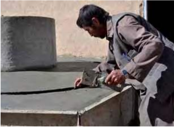
Construction of water well in Malistan, Ghazni
