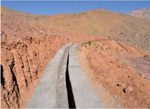
Irrigation canal built in Malistan, Ghazni
