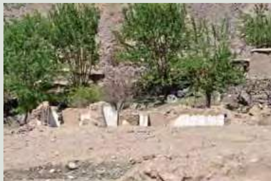
Abdul Rahman's house which was destroyed
