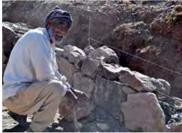
During the construction of an irrigation canal in Malistan
