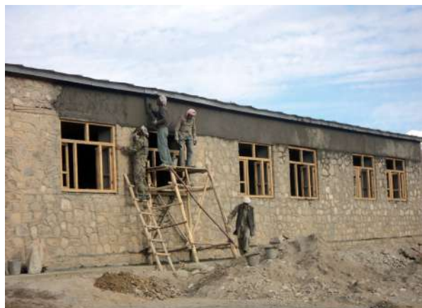
Madena School Renovation
