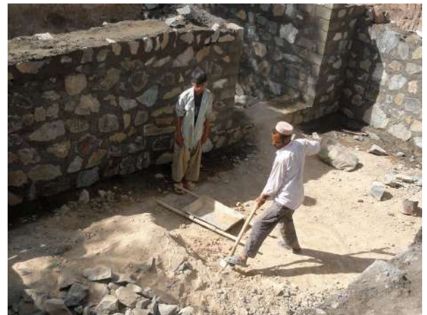
Cold Store Construction in Shahr-i-Wahdat
