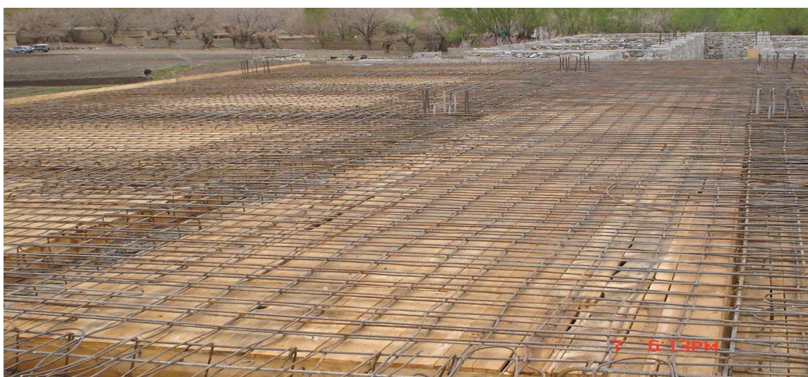
Tir Garan girls' school, construction initiated in 2007 to be completed in 2008
