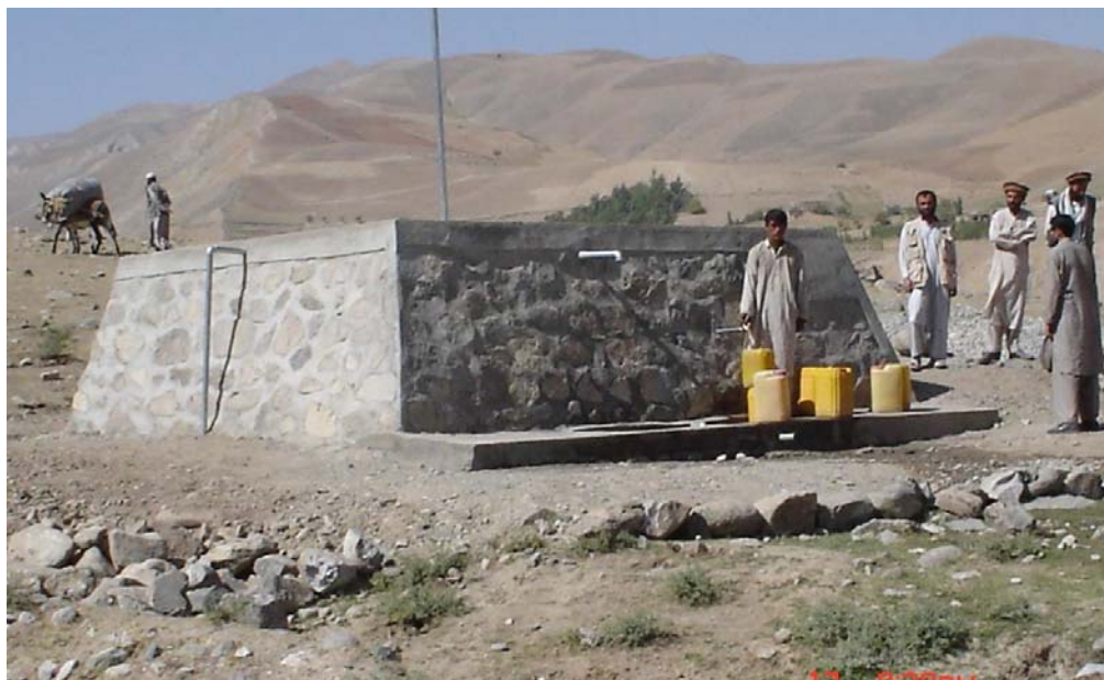
Water reservoir in Koshem Dara Yaftal district, Badakhshan province
